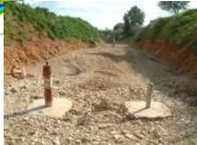
3) Carreiros test site 2 Infiltration basins in the river bed
